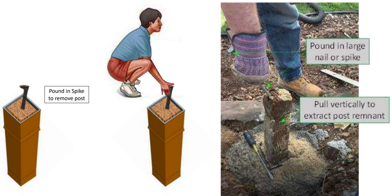
Figure R2c. Shows post with nail or spike protruding from post end to grasp and pull out of ground
