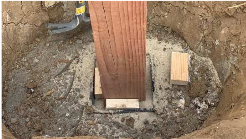
Figure 5c. Placing locking shim blocks
