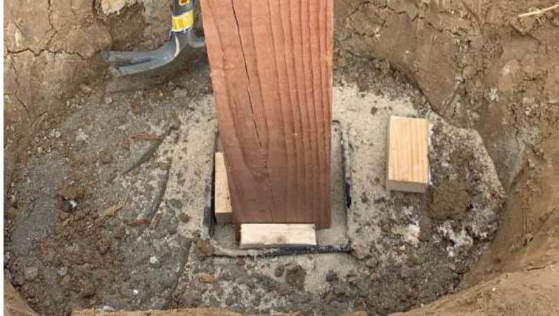
Figure 5c. Placing locking shim blocks
