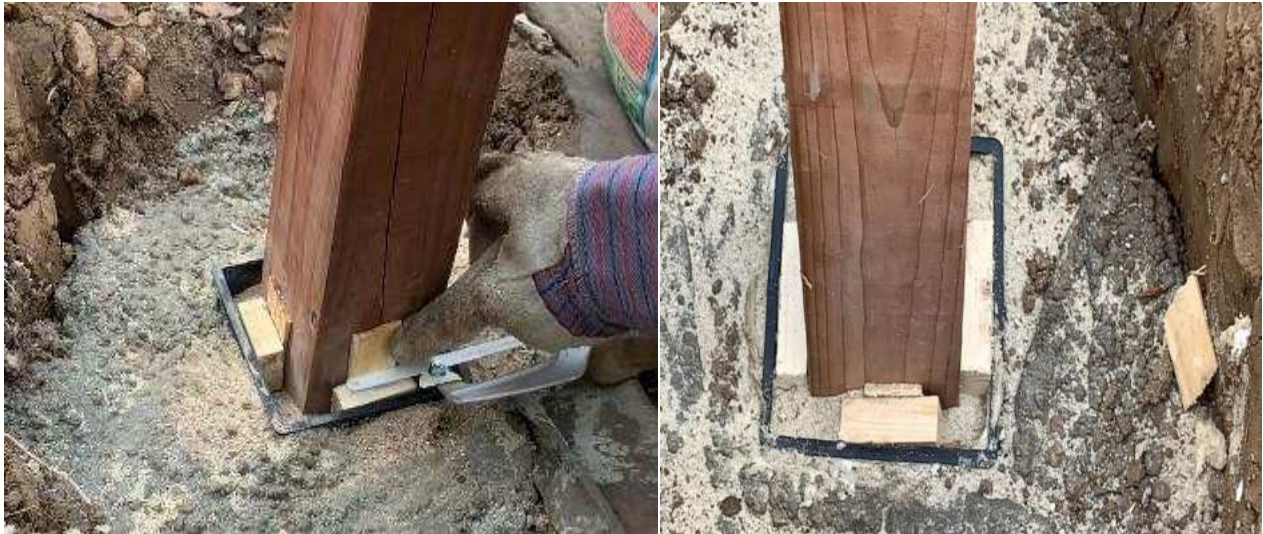
Figure 5e. Scoring and breaking off the door shims
