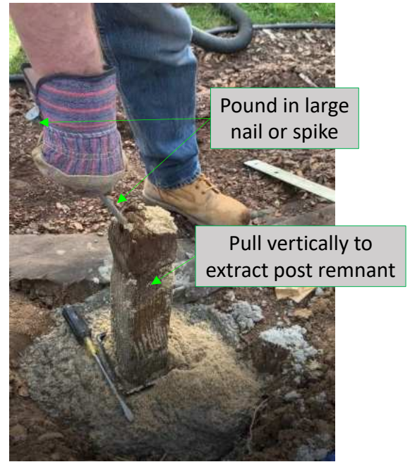
Figure R2c – shows post with nail or spike protruding from post end to grasp and pull out of ground
